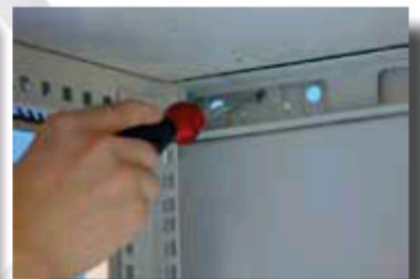
Inside fixation by nuts to avoid accident
